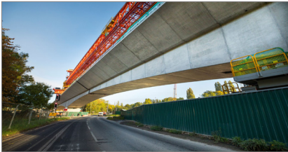
Completed A412 road crossing between P55 and P54 with a grout connection at the Colne Valley Site, October 2022
