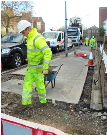
Colas Ltd's maintenance team resurfacing the pavement
